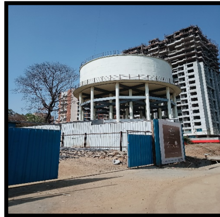
Construction of Elevated storage Reservoir near project site
